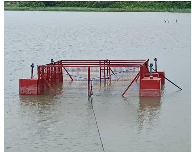
Fig. 12: The developed semi-submersible offshore fish farm moored in a Nigerian inland water.
